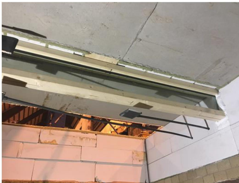
Fig. 4: Photo during setup of the beams before testing
