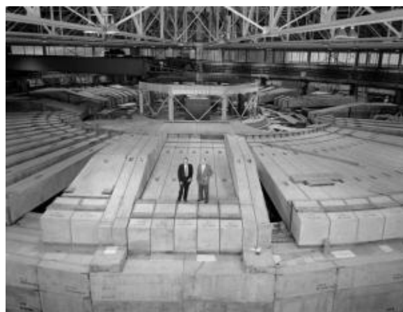
Fig. 28: Edwin McMillan and Edward Lofgren on the shielding of the Bevatron. The shielding was only added later, after initial operations
