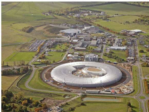
Fig. 32: Aerial view of The Diamond Synchrotron
